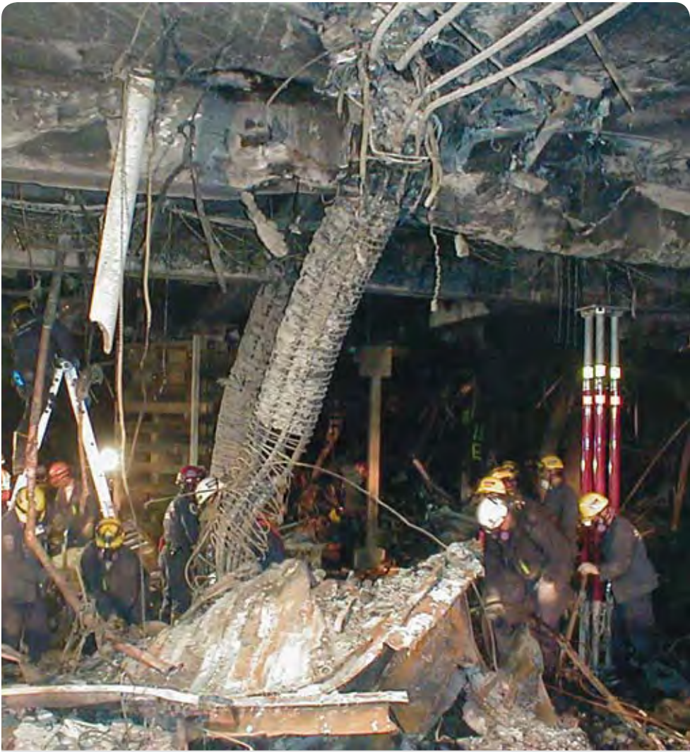
Airshore strut systems in operation: Pentagon, September 2001, US & R teams.
