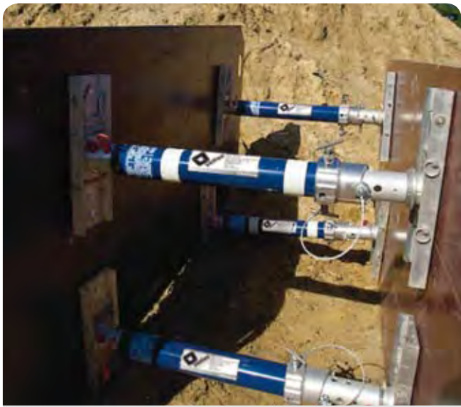
Trenches can also be safely supported with Airshore.
